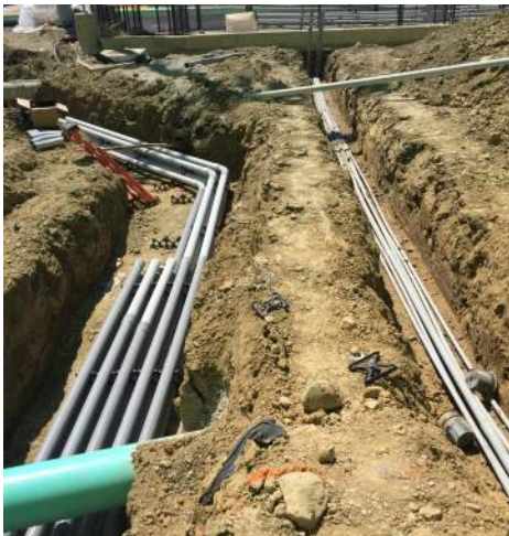
Area A Electrical Duct Banks
