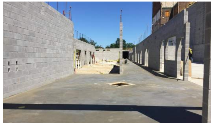
Area C Slab-On-Grade
