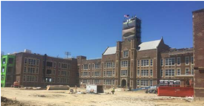
Courtyard & Clock Tower Restoration
