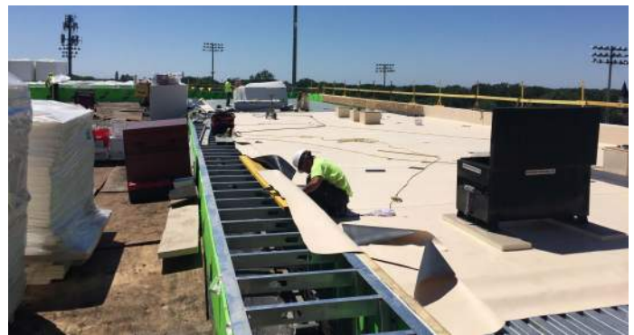
Area A Existing Roof Demo (left side) & New Roof Installation (right side)
