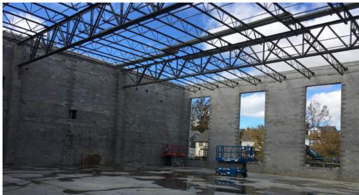
Auxiliary Gym Area C Washington Level
