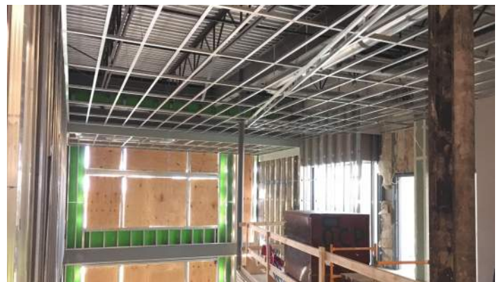
Area A Atrium Ceiling Framing
