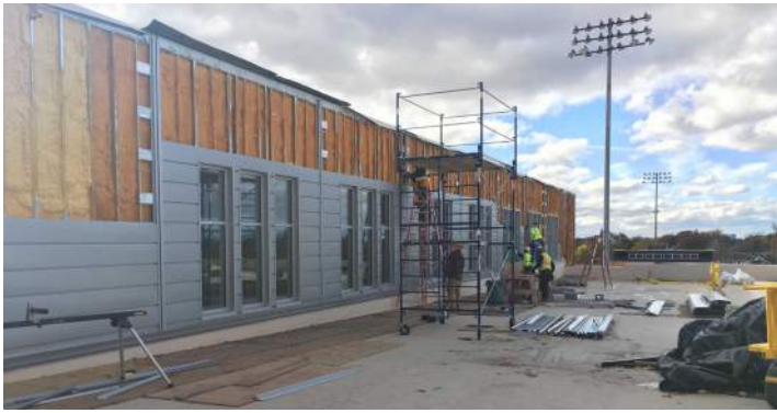
Metal Veneer Panels Area A North Elevation 3rd Floor
