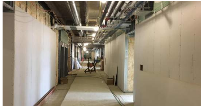
Area G 3rd Floor Corridor
