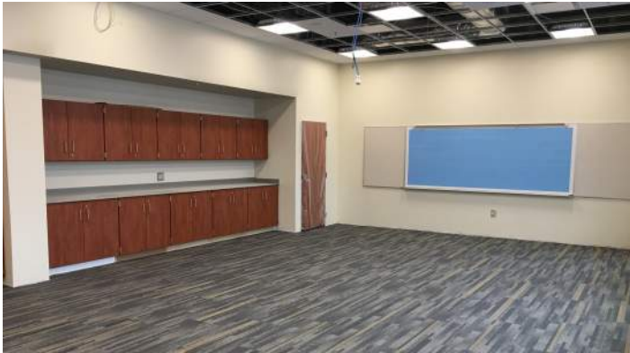
Carpet Tile Installation Area A 3rd Floor
