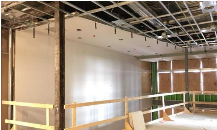
Gypsum Board Installation Area A 3rd Floor
