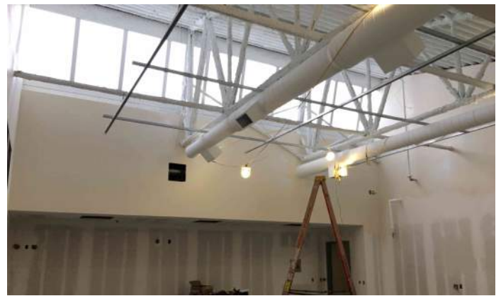
Science Classroom Duct & Ceiling Painting Area E 2nd Floor
