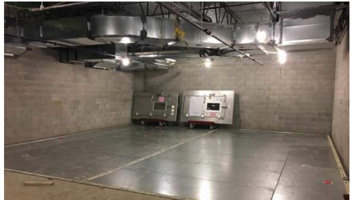
Walk-In Cooler Installation Area D Washington Level
