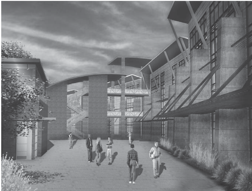
V. Sue Cleveland High School: The new V. Sue Cleveland High School in Rio Rancho, New Mexico, features an energy-efficient façade with light shelves that shade lower window areas and transfer natural light through the upper windows into the classrooms. (Design team of Fanning Howey and Van H. Gilbert Architects)
