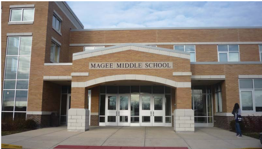
Left: Magee Middle School was one of nine buildings that received a complete assessment and educational adequacy analysis.
