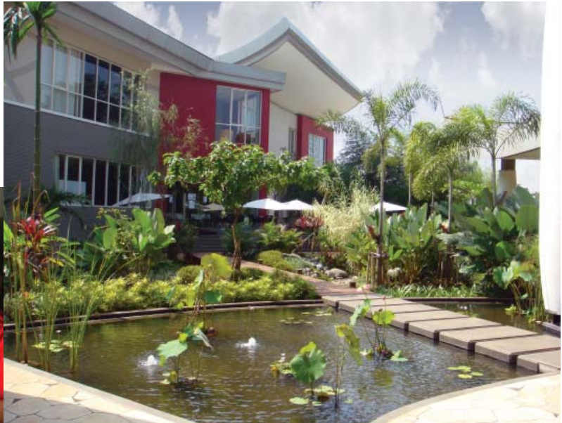
Above: Gardens and a pond serve as learning opportunities for Sinarmas students - note the large over-hangs that shade the windows and doors from the intense local sunlight
