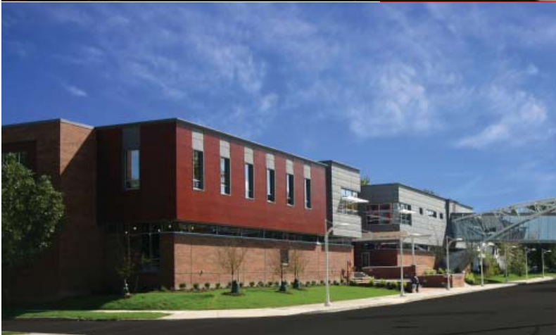
Above: Exterior building views showing the landmark pedestrian walkway that serves as a place for kids to race each other as well as specifically choreographed dance exhibitions.
