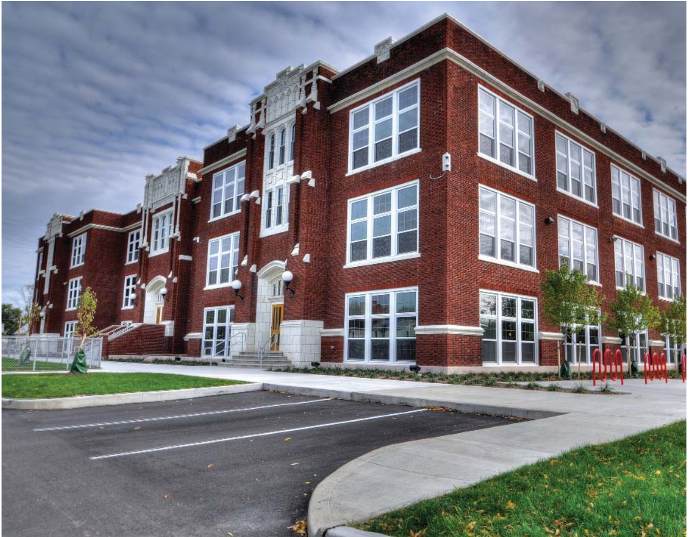
Above: The building's historic main entrance was preserved, but behind its walls lies a 21st century learning environment.
