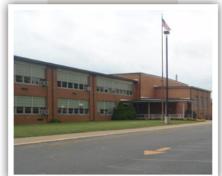
Southern Local High School Addition Racine, OH
