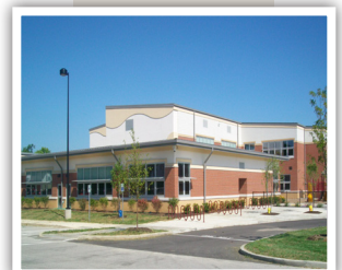
Edgerton School Expansion Edgerton, OH
