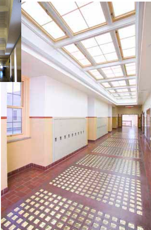
BEFORE AND AFTER PHOTOS Ceiling
