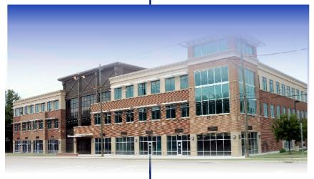
The steel frame and exterior metal stud walls with brick, cast stone and veneer was designed for LEED Silver certification. The aluminum windows and curtain walls will deliver a lot of natural light into the interior spaces and contribute to achieving LEED goals.
