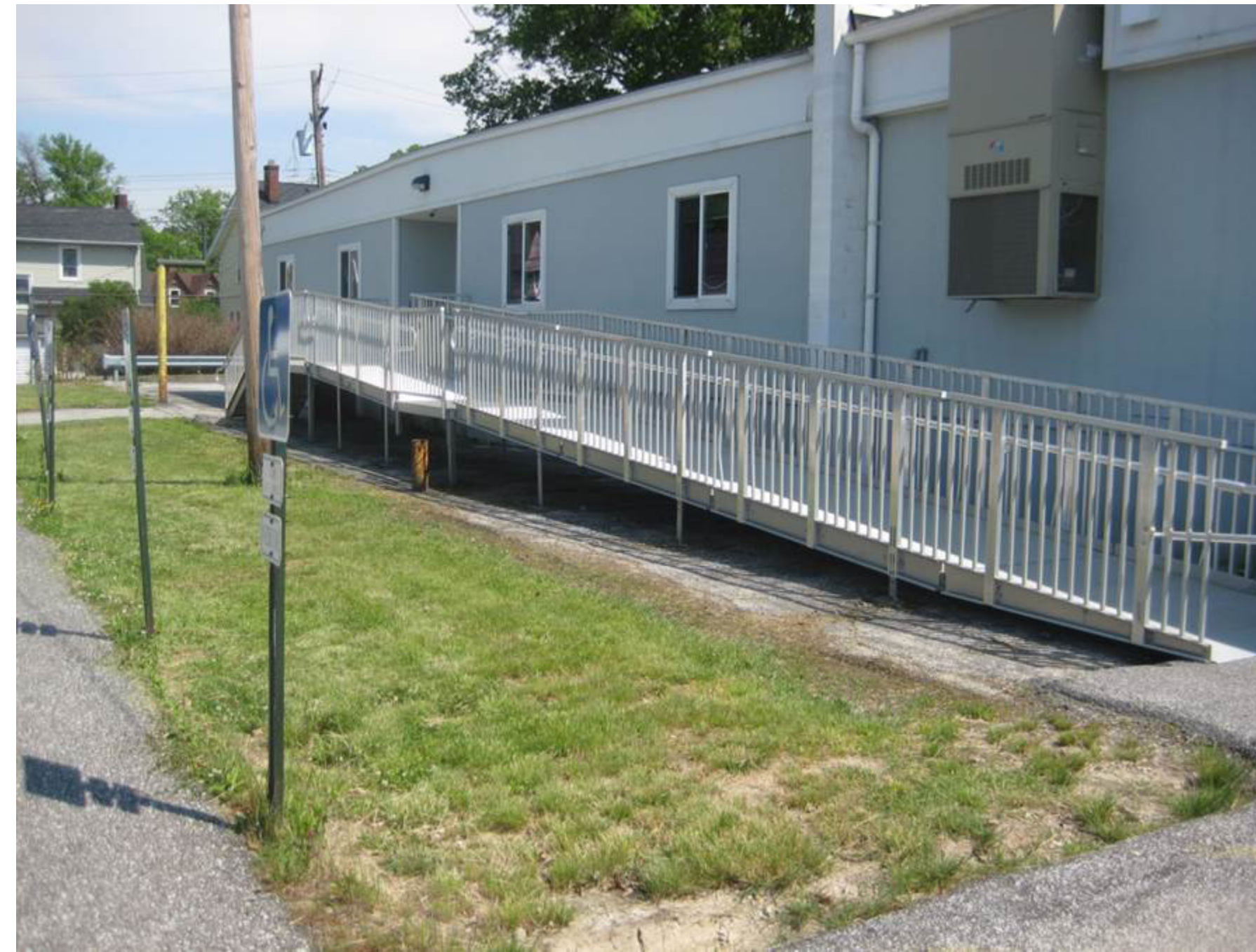
Exterior Entrance with Ramp
