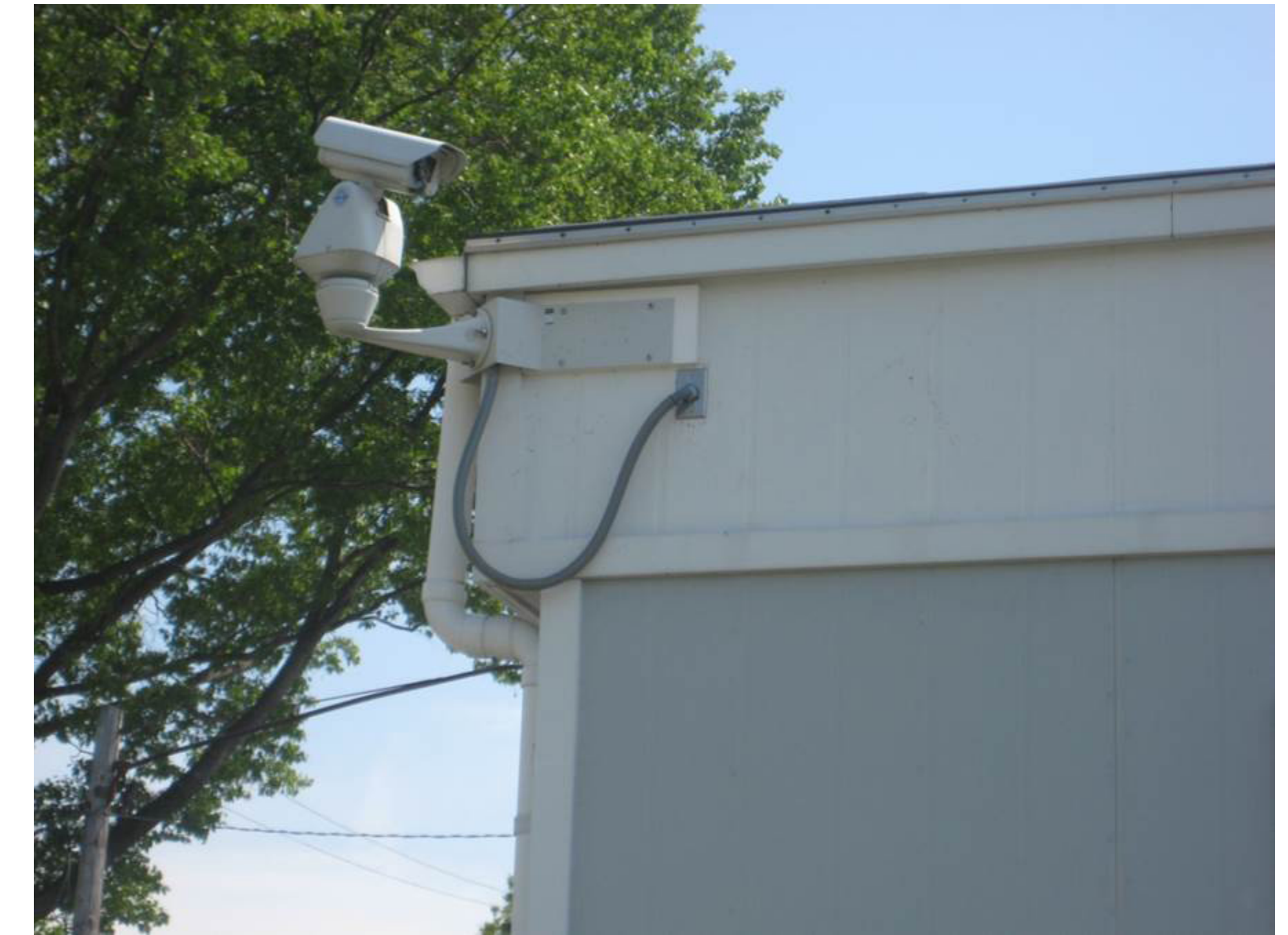
Exterior Security Camera
