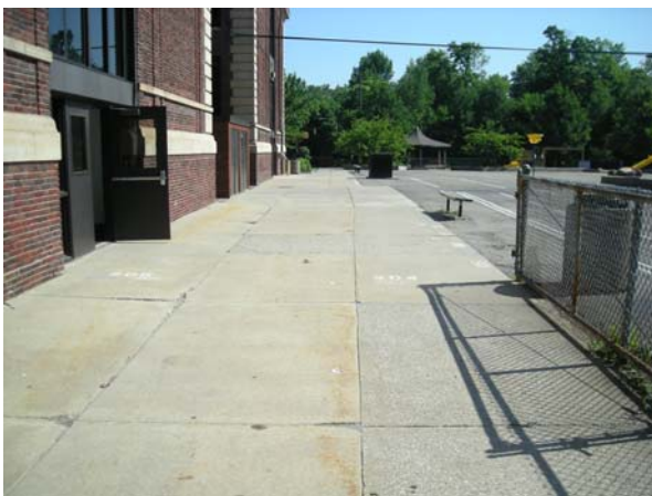
Concrete paving at rear of building
