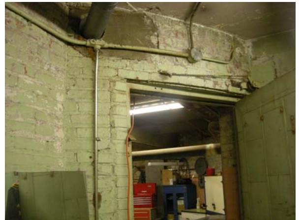
Boiler room wall
