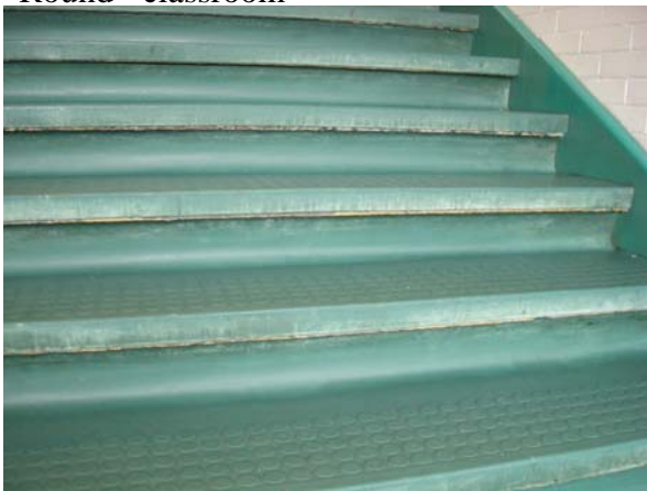
Typical riser and tread condition
