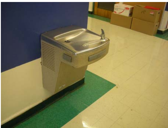
ADA Compliant drinking fountain
