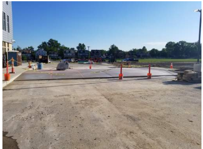
Constructing East Crosswalk
