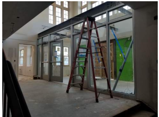
Framing Area C Vestibule
